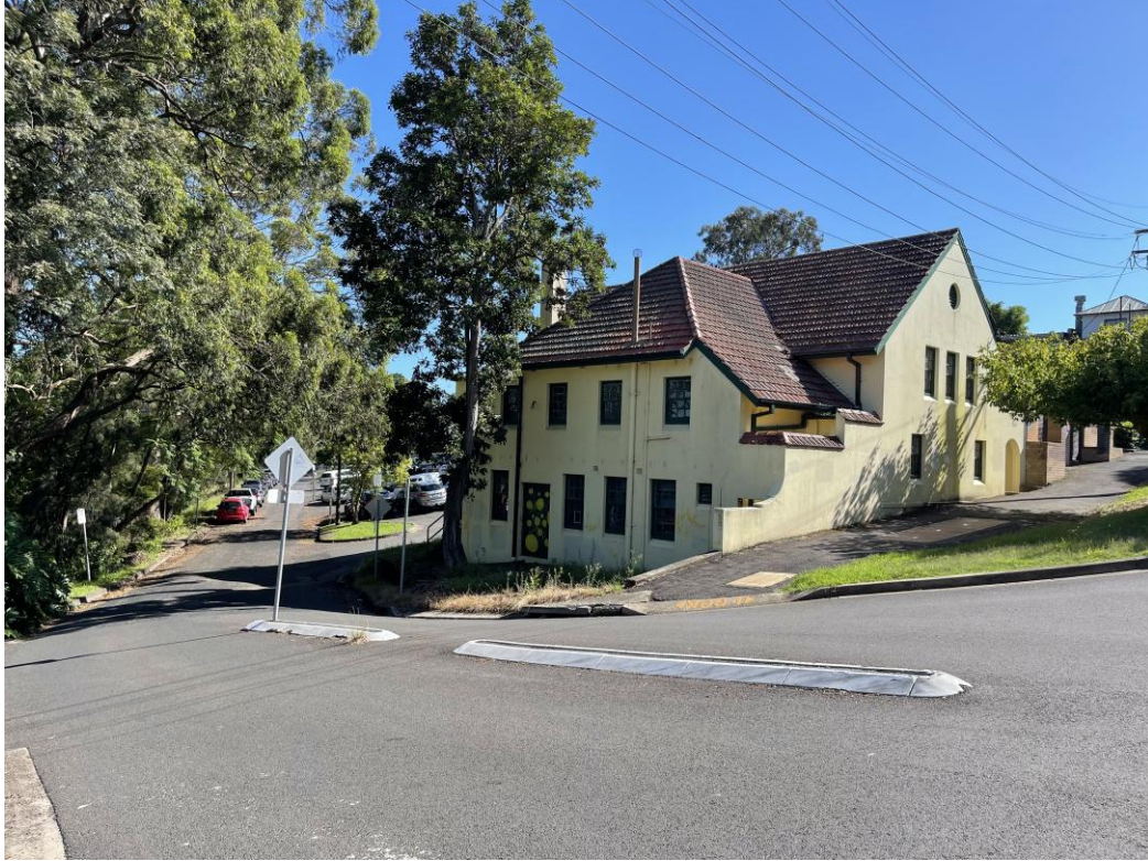
Fig 8: View of the adjacent Lindfield Village Hub commercial area, looking north from Beaconsfield Parade
