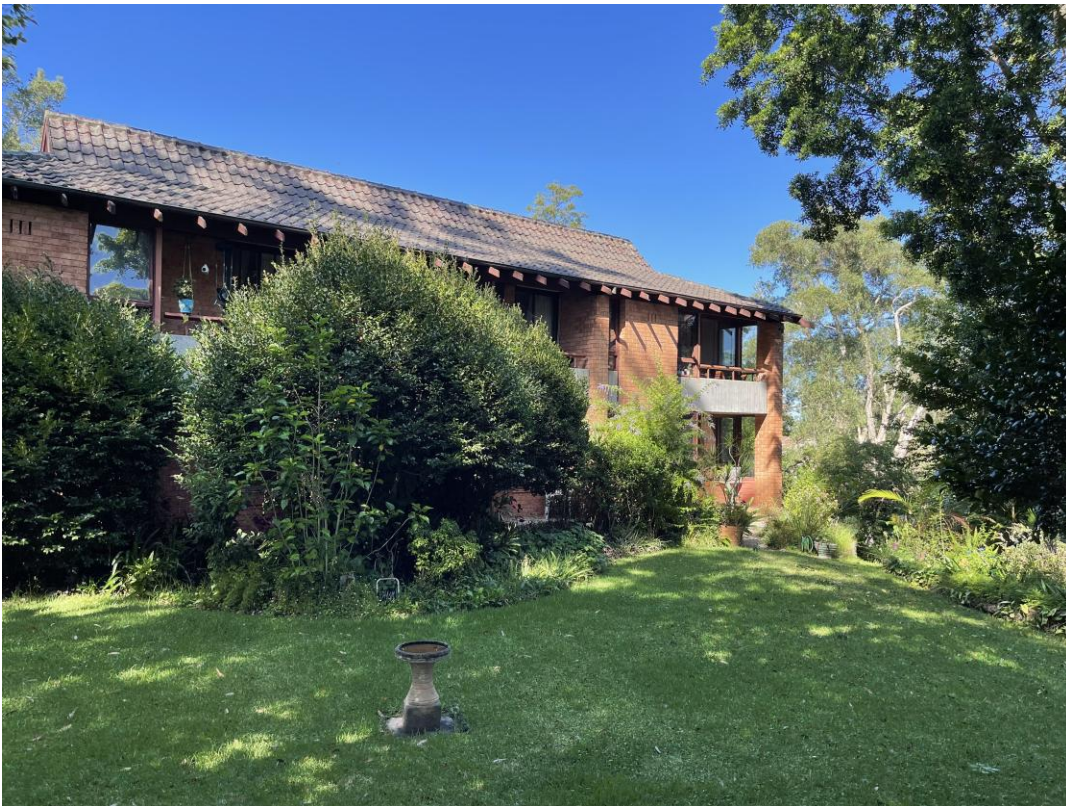
Fig's 10 & 11: Views of the existing medium density development within No 3 Beaconsfield Parade, looking south and south-west respectively
